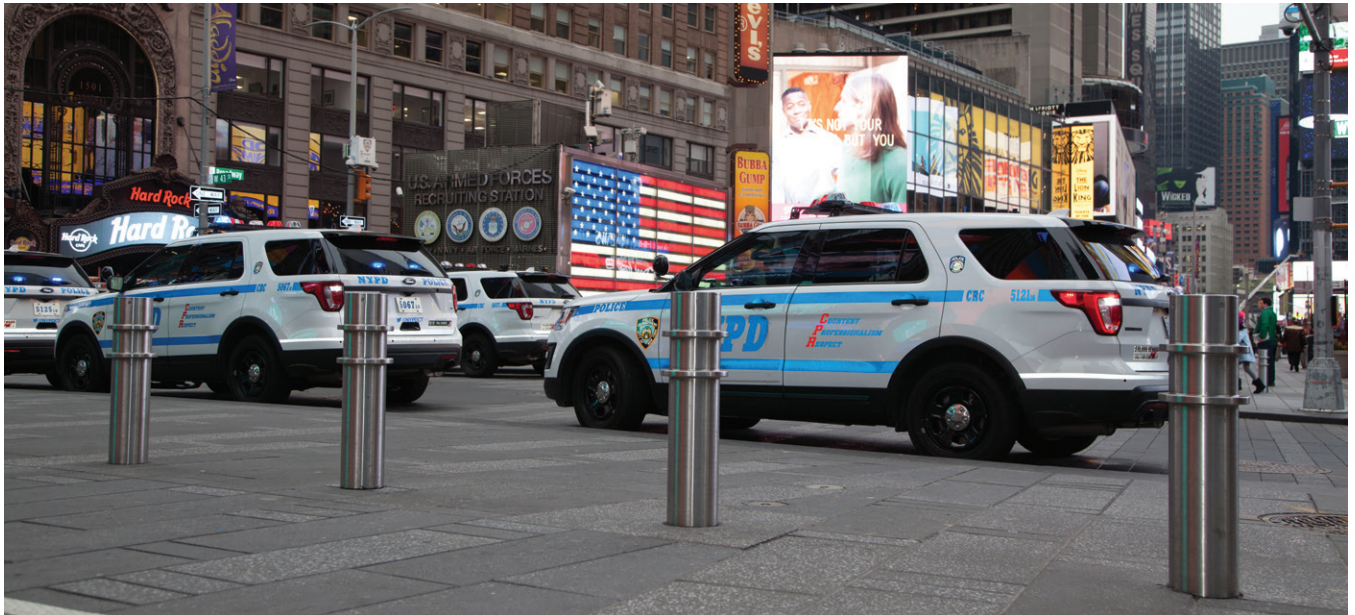
Times Square in New York is now protected by crash-rated removable bollards. Improving security at a public space or commercial storefront also provides greater safety to the public and invitees as well. (Photo: Calpipe Security Bollards)
